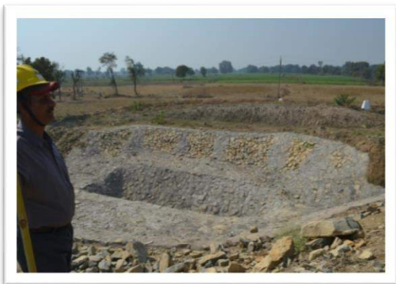
Garland DrainSettling Pond
