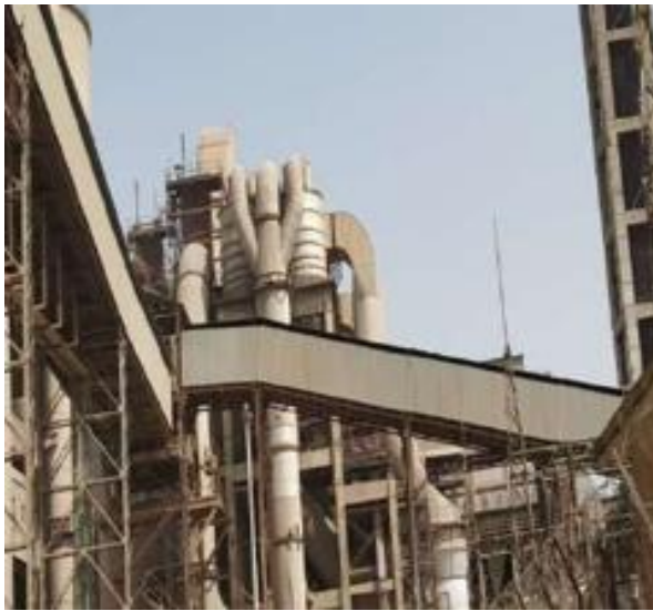
Covered Conveyor Belt & Bag filters
