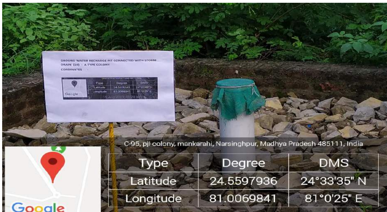
RWH 10 – Ground Water Recharge pit connected with Storm Drain Near A type colony
