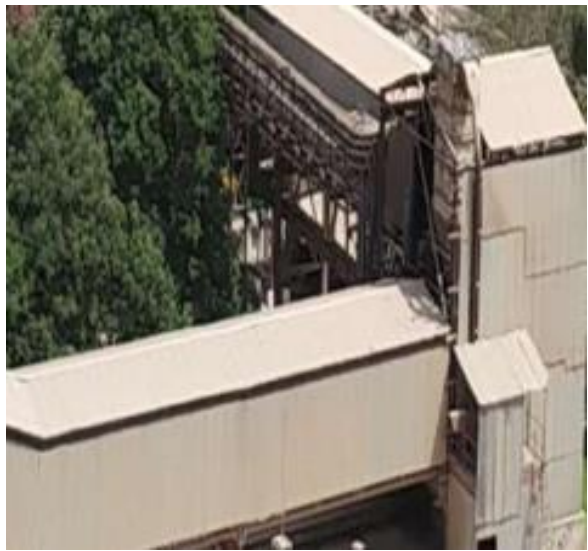
Covered Conveyor Belt & Bag filters
