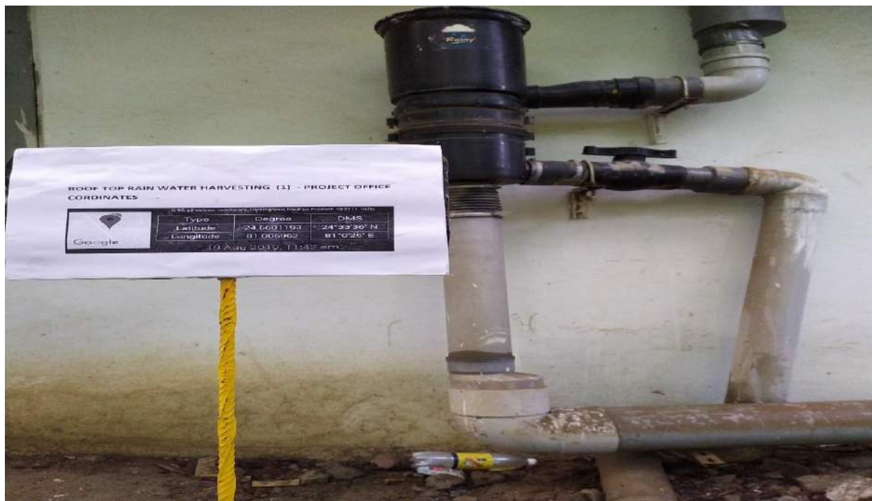
RHH 1 – Roof top Rain water Harvesting - Project Office
