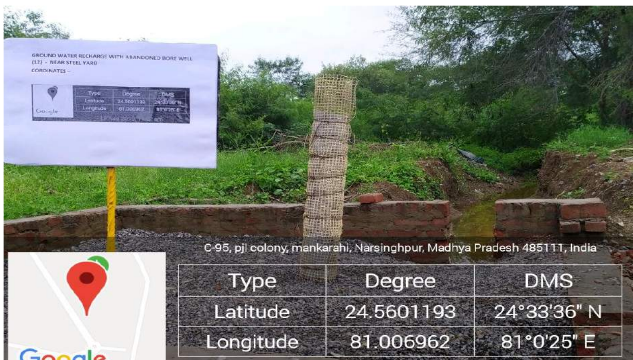
RWH 12 - Ground Water Recharge pit with abandoned Bore well – Near steel yard
