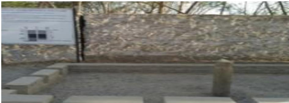
**4. Construction of Percolation Tank with Bore Holes:** A big percolation tank of size 46.5 X 3.5 X 1.5 Meter is made with four numbers of boreholes. Perforations made in the casing inside recharge structure and wrapped with fine net. Excavated pit has been filled with conventional filters.
