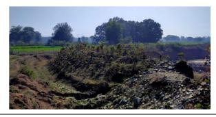
Top soil / solid waste shall be stacked properly with proper slope and adequate safeguards and shall be utilized for backfilling (where ever applicable) for reclamation and rehabilitation of mined out area. Top soil shall be separately stacked for utilization later for reclamation and shall not be stacked along with over burden.
