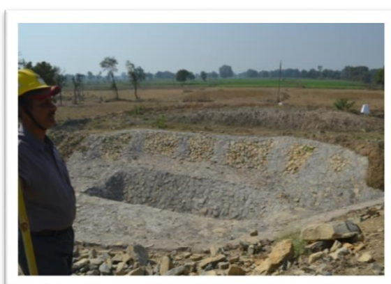
Garland DrainSettling Pond
