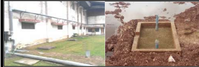
Artificial ground water recharge structures
