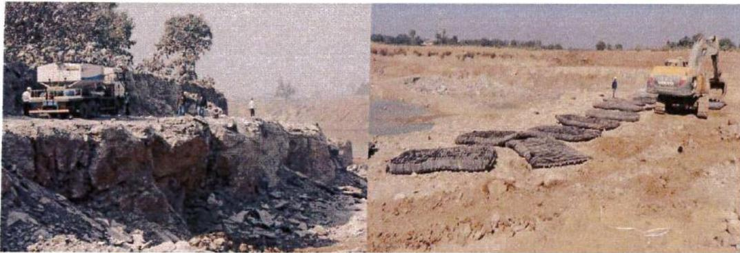
Photograph 2. The charging of the 15 no. RPL bench and use of blasting mate at 7050 RIL blast face to prevent flyrock.
